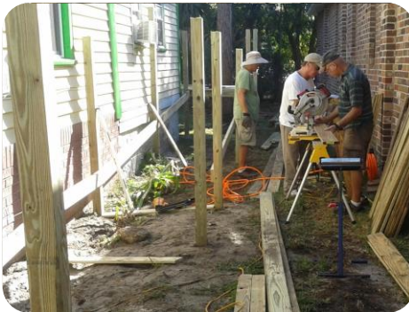
Building Ms. Bertha's New Ramp
