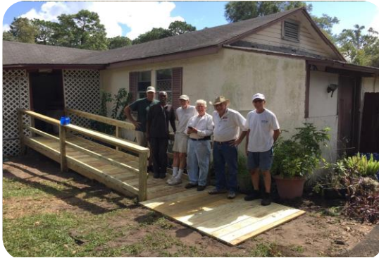
Ramp-building Team and Mr. Ben's New Ramp
